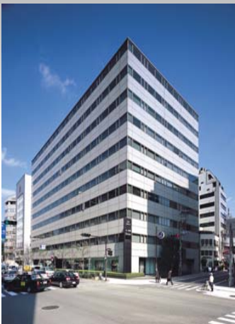
II-2 JEI Nishi-Honmachi Building
