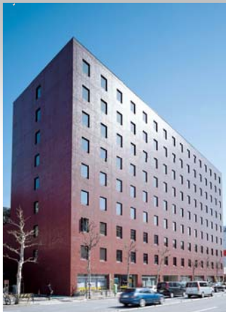
I-4 No.32 Kowa Building
