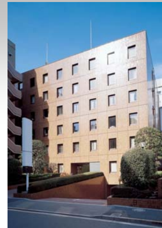
I-5 No.36 Kowa Building
