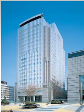
II-1 NHK Naoya Housou-Center Building
