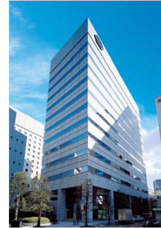
I-2 Shiba 2-Chome Building
