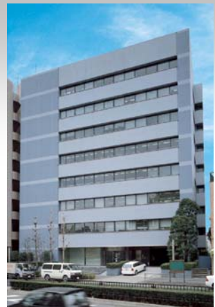
III-3 JEI Hongo Building
