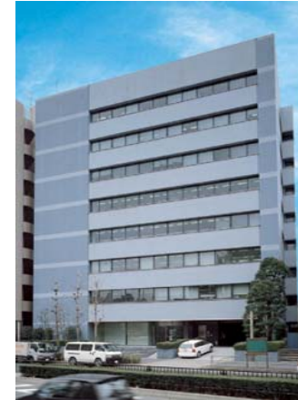
III-3 JEI Hongo Building
