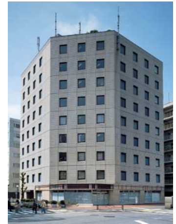
III-6 No. 44 Kowa Building
