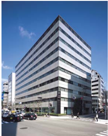
II-2 JEI Nishi-Honmachi Building
