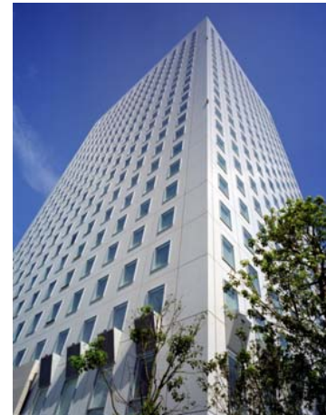
III-8 Ebina Prime Tower
