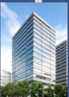
Kowa Nishi-Shimbashi Building 1997
