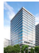
Kowa Nishi-shimbashi Building
