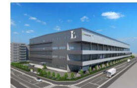
LOGIFRONT Koshigaya I (logistics) Scheduled for completion in February 2019
