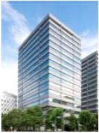
Kowa Nishi-Shimbashi Building
