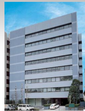
III-3 JEI Hongo Building
