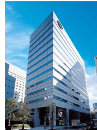
I-2 Shiba 2-Chome Building
