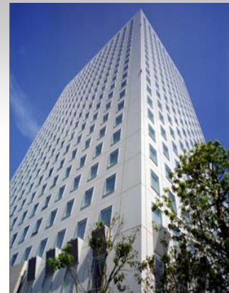
III-8 Ebina Prime Tower
