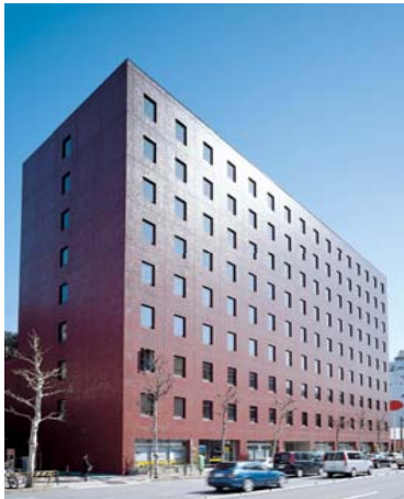
I-4 No. 32 Kowa Building
