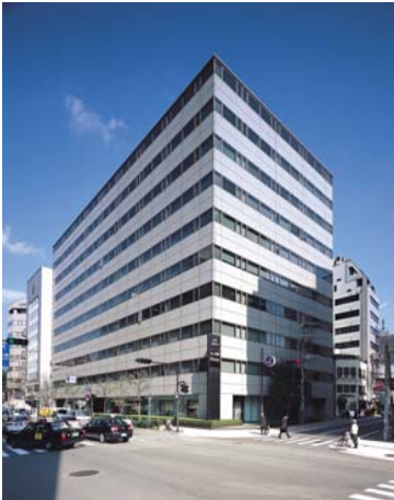
II-2 JEI Nishi-Honmachi Building
