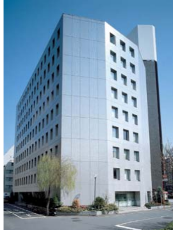
I-6 No. 28 Kowa Building
