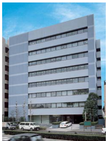
III-3 JEI Hongo Building
