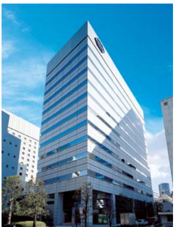
I-2 Shiba 2-Chome Building
