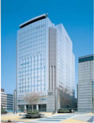
II-1 NHK Naoya Housou-Center Building
