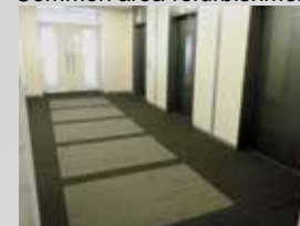
Kawasaki Nisshincho Building Common area refurbishment
