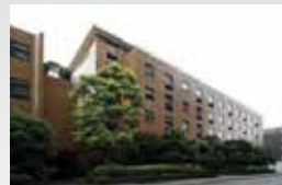
No. 35 Kowa Building
