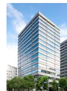
Kowa Nishi-Shimbashi Building
