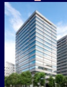
Kowa Nishi-Shimbashi Building 1997
