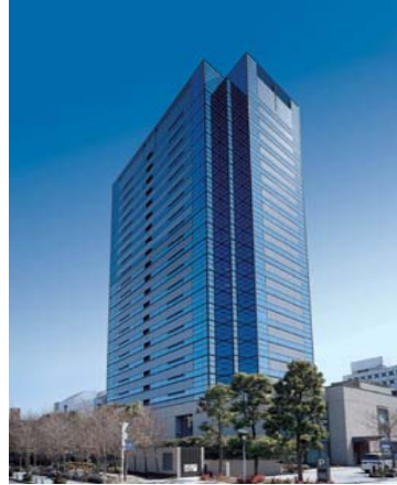
III-1 Musashikosugi Tower Place
