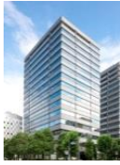
Kowa Nishi-shimbashi Building
