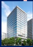
Kowa Nishi-Shimbashi Building 1996
