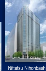
Nittetsu Nihonbashi Building 2019
