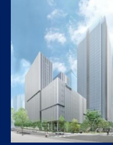
Toranomon 2-Chome Redevelopment Scheduled for completion in November 2023
