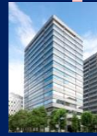
Kowa Nishi-Shimbashi Building 1996
