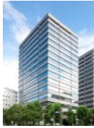
Kowa Nishi-shimbashi Building
