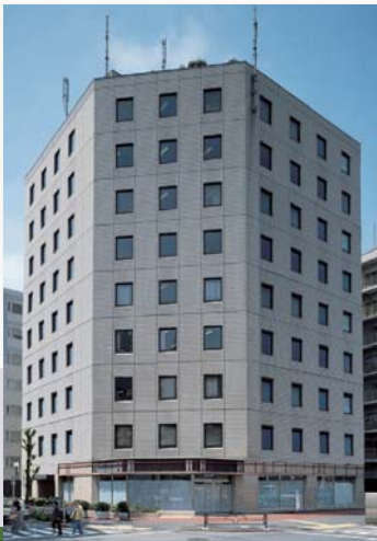
III -6 No. 44 Kowa Building
