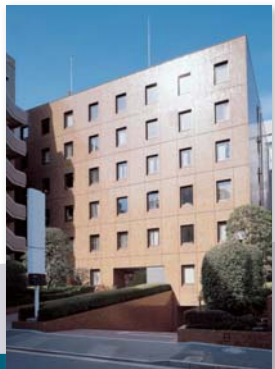
I -5 No. 36 Kowa Building
