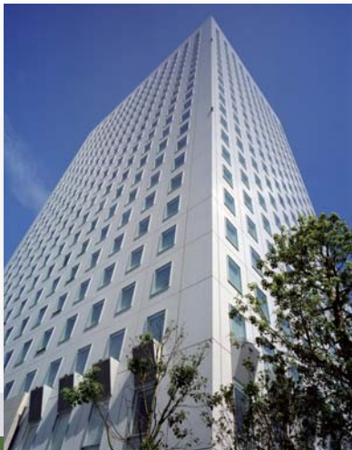
III -8 Ebina Prime Tower
