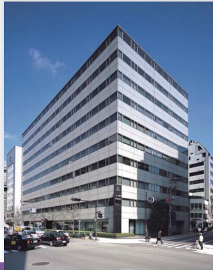
II -2 JEI Nishi-honmachi Building
