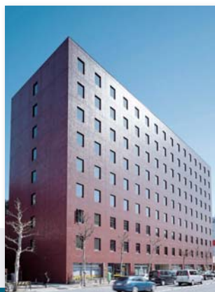
I -4 No. 32 Kowa Building
