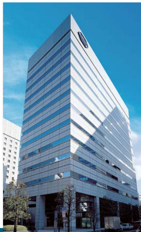
I -2 Shiba 2-Chome Building
