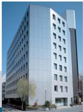
I -6 No. 28 Kowa Building
