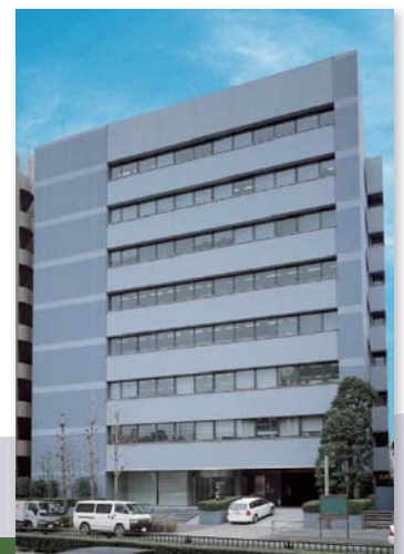
III -3 JEI Hongo Building
