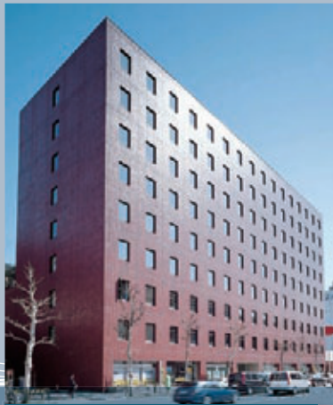
I-4 No. 32 Kowa Building
