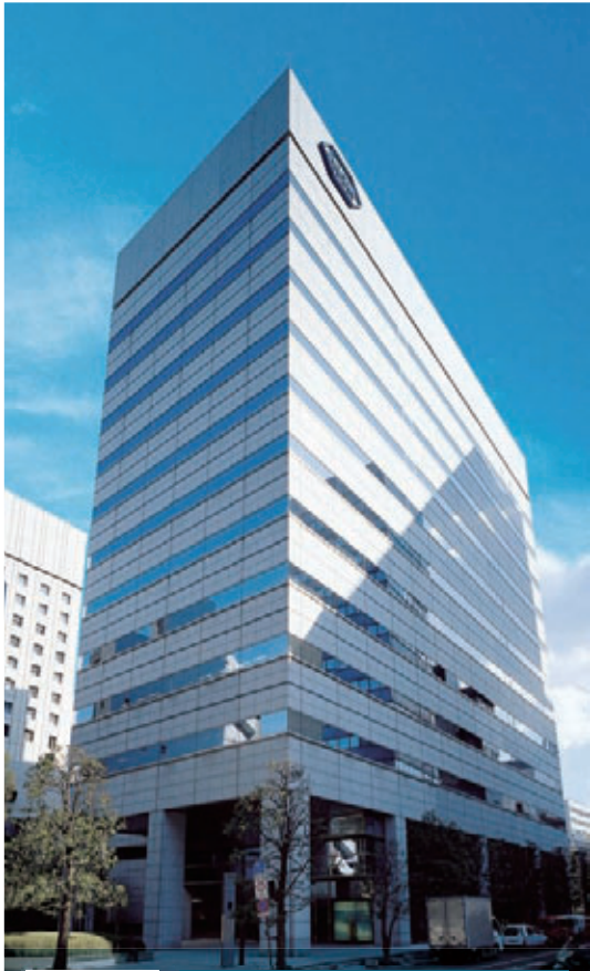
I-2 Shiba 2-Chome Building
